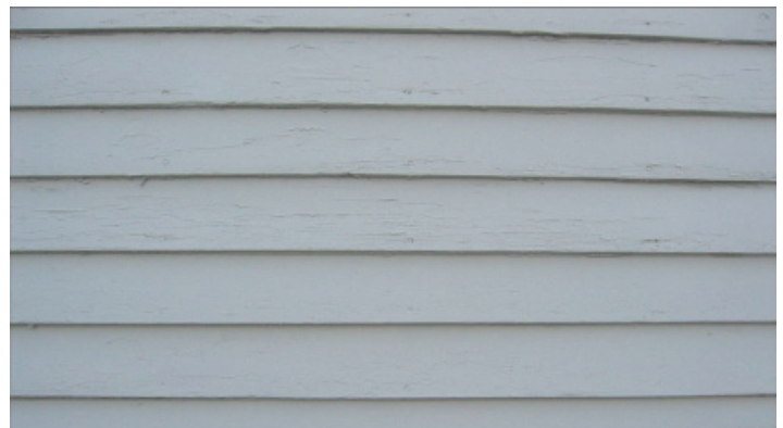
Horizontal boards that are flat or beveled are referred to as weatherboard and are common to a wide variety of architectural styles.
