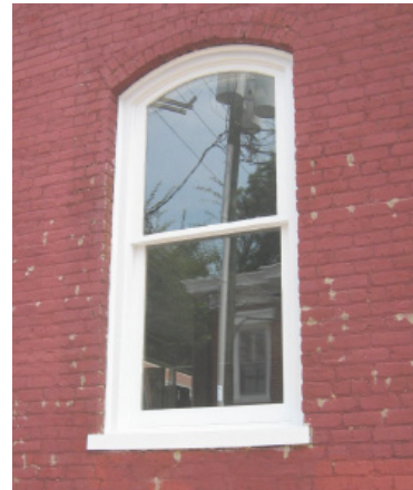
One-over-one with segmental brick arch.
