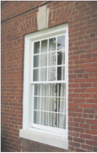
Twelve-over-twelve with keystone and brick flat arch.
