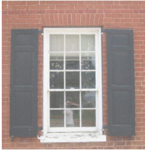
Nine-over-six with operable shutters and jack arch.
