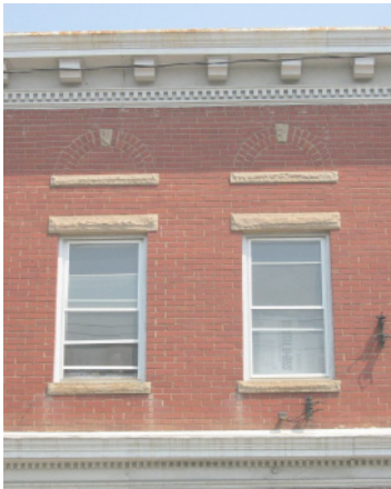
One-over-one with rough faced stone lintel.
